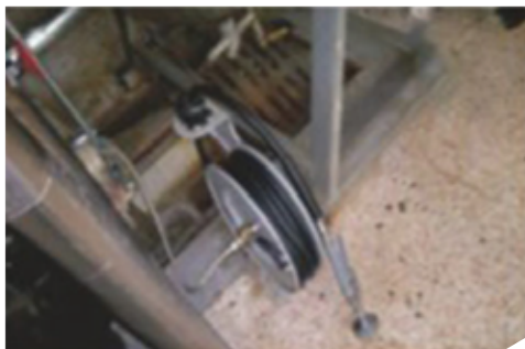
It is forbidden to install underground to affect water pressure and stretch recovery.
